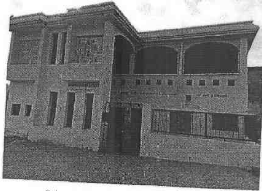
School constructed in Chotti Badi Naggal
