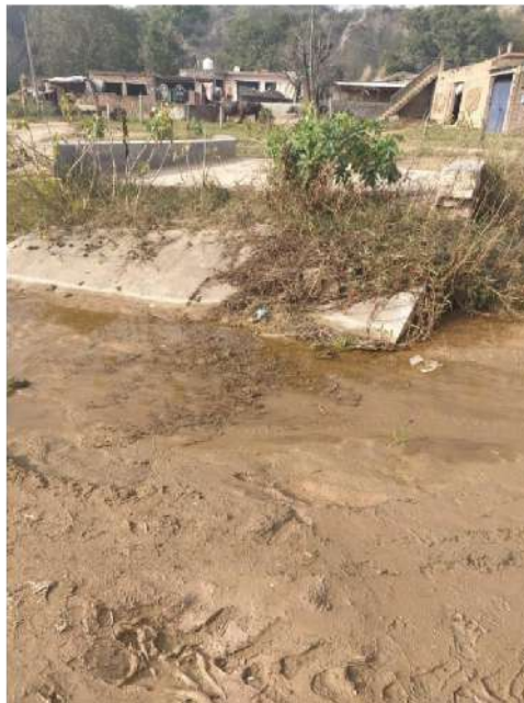
Bridge constructed in Chotti Badi Naggal
