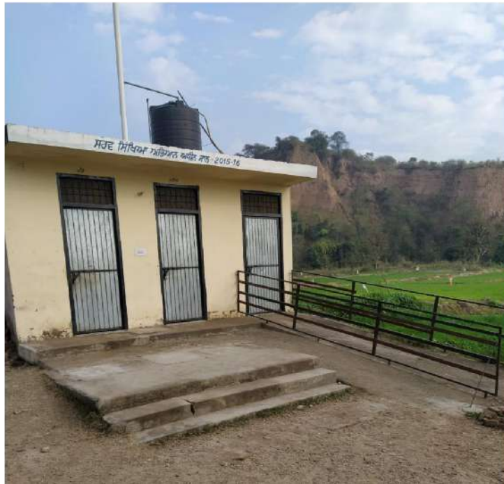
Toilets constructed in Chotti Badi Naggal
