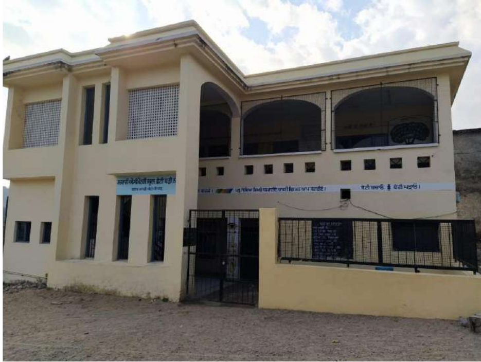
School constructed in Chotti Badi Naggal
