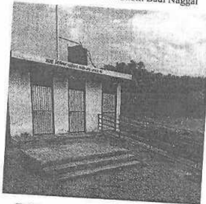
Toilets constructed in Chotti Badi Naggal
