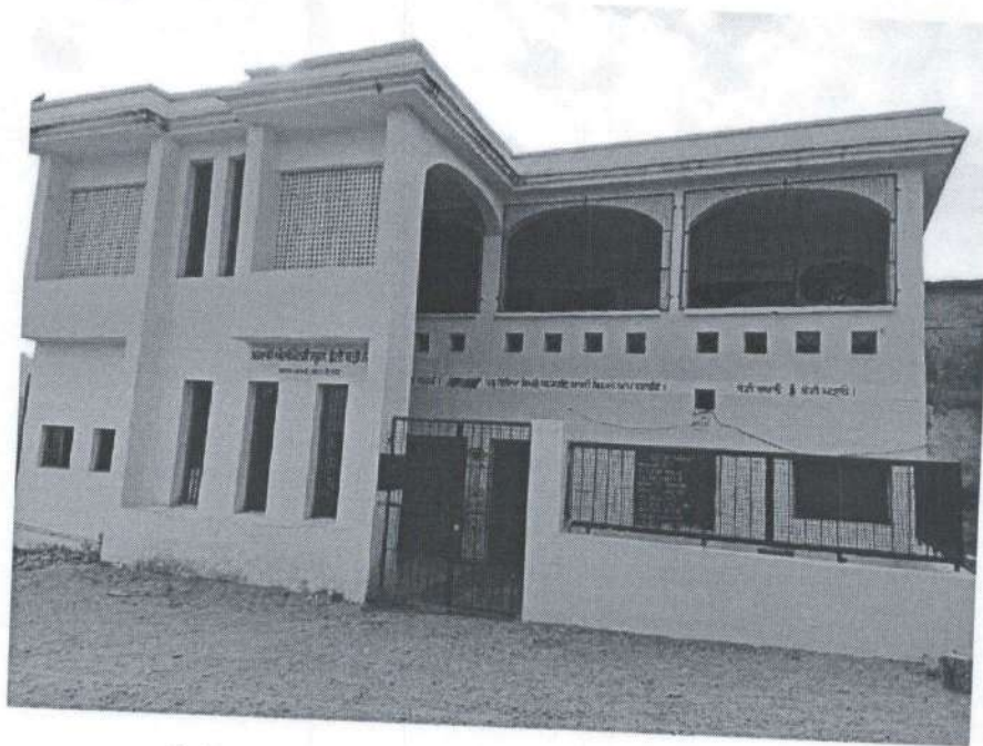
School constructed in Chotti Badi Naggal
