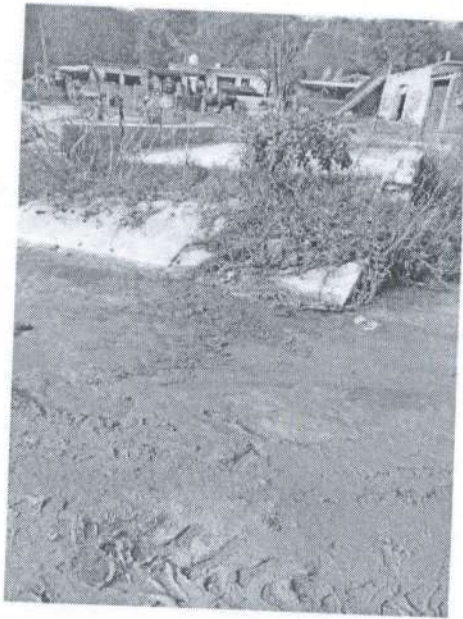
Bridge constructed in Chotti Badi Naggal
